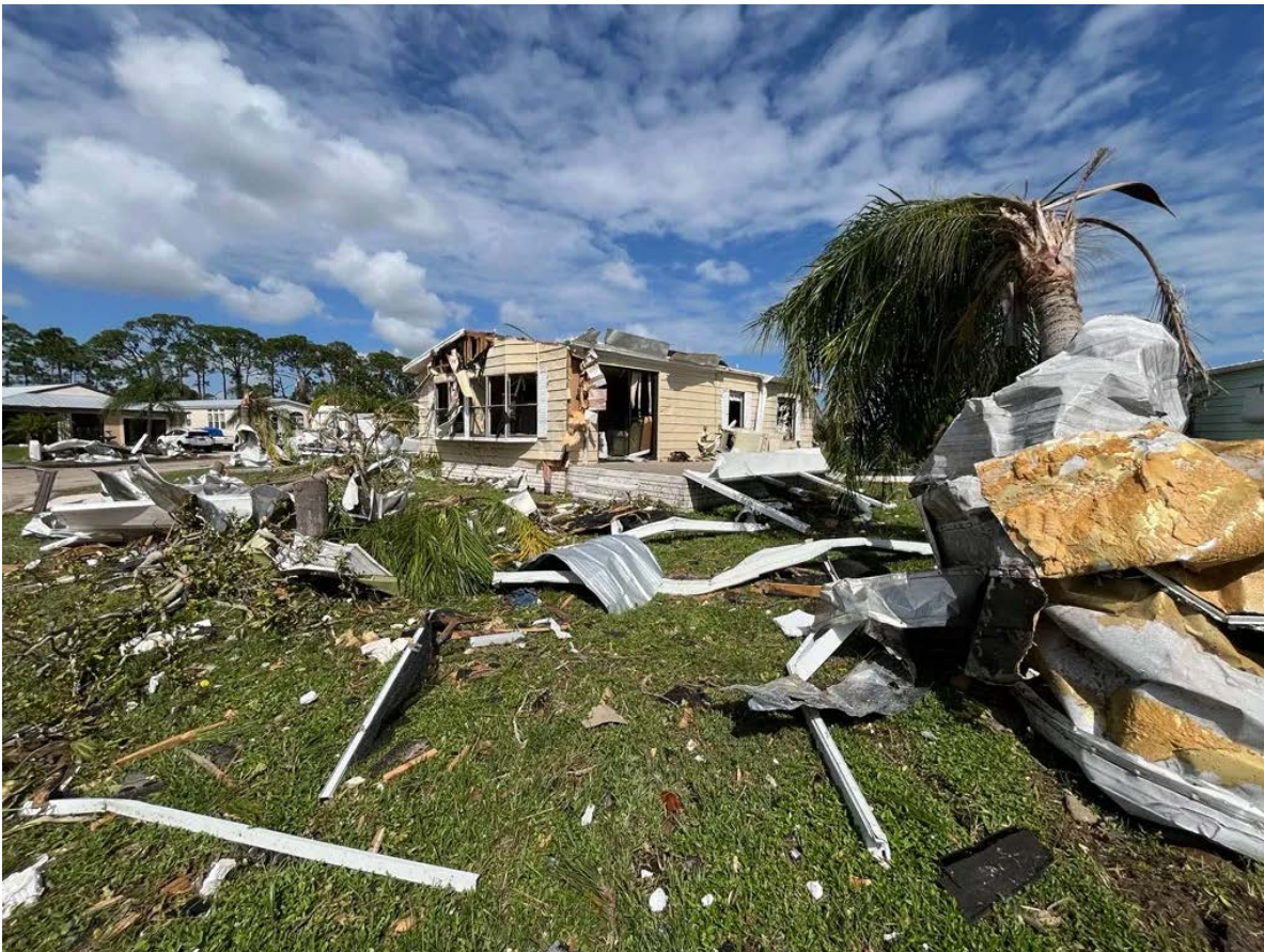
Damage from Hurricane Milton in Fort Pierce, Florida (credit: FEMA, Patrick Moore).
