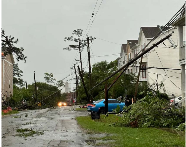
Damages from tornadoes, May 10, 2024, in Tallahassee (source: Tallahassee Democrat).
